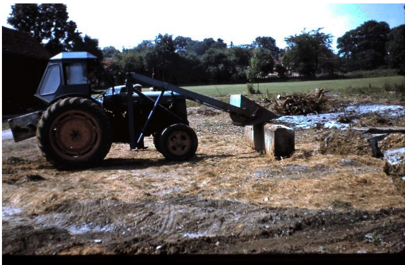
Clearing the concrete bases
