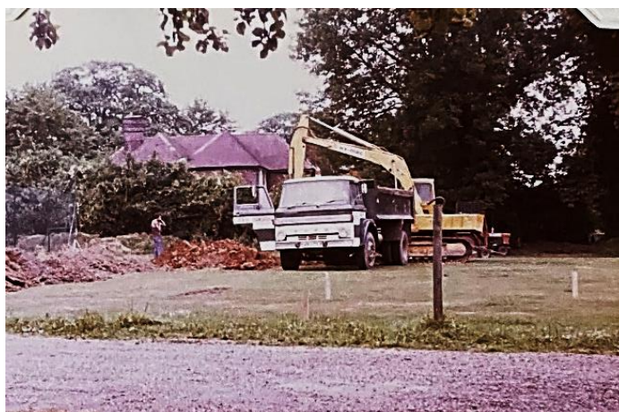
Work starts on building the swimming pool
