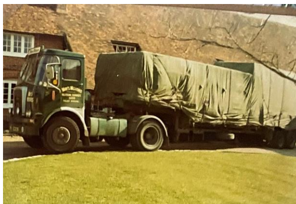
The lorry delivering the Guildway Building
