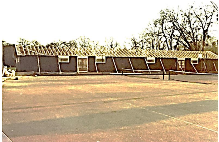
Work continues on the new Winterbourn building
