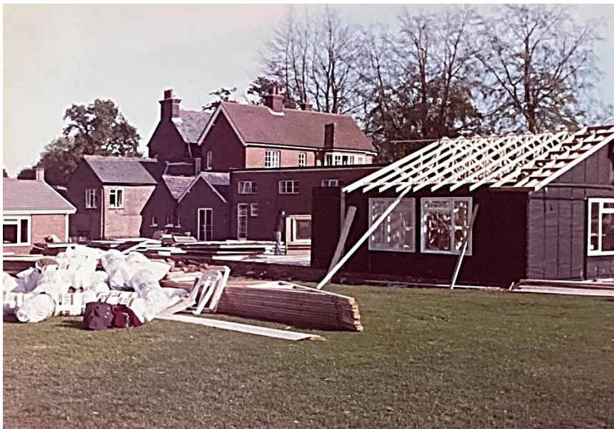
Work in progress on the Jones Building
