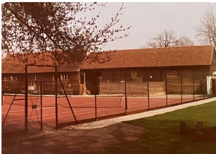
The new En Tout Cas tennis courts with PLM’s protective measures for the netting
