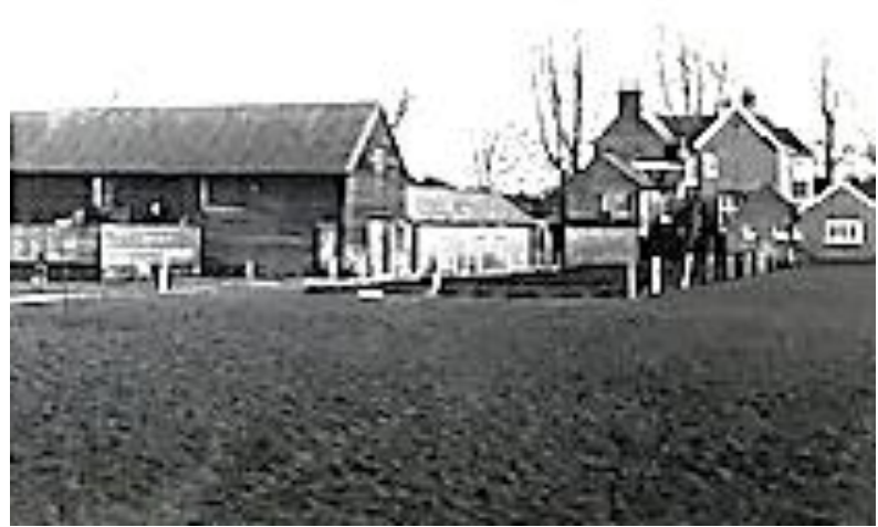
The site for the Strong Building
