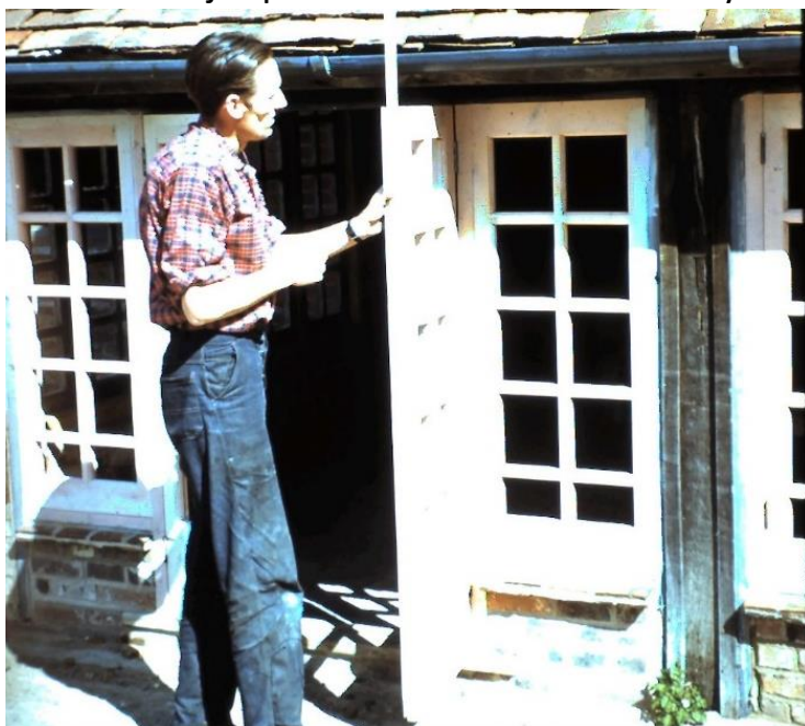
Jim Ross, carpenter, working on the front of the headmaster's house
