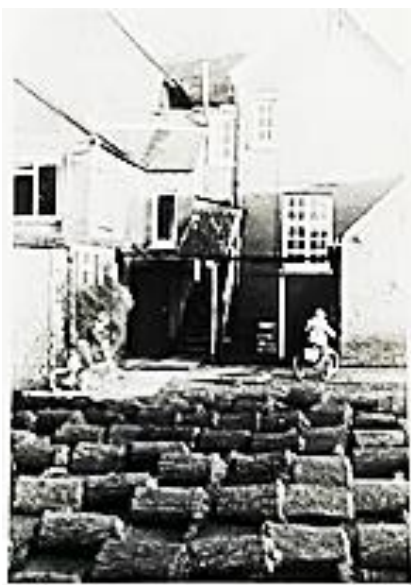
Stripping the turf
