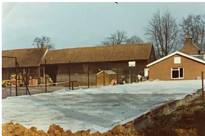
Work started on the new Winterbourn building in May 1977
