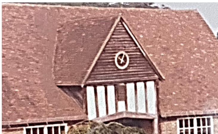
The new clock on the gable installed 24 May 1961
